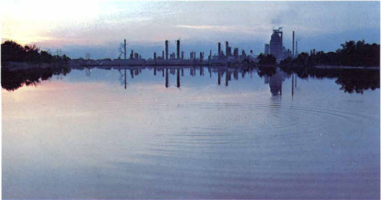
Phillips Petroleum's refinery at Sweeny, Texas.
