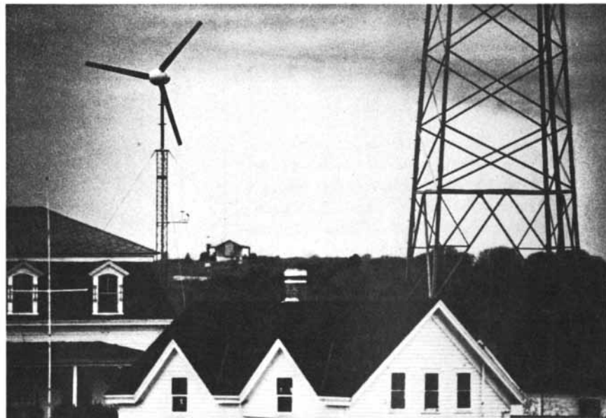
Windmill helps power central phone office and microwave radio terminal (tower at right) on Block Island.
