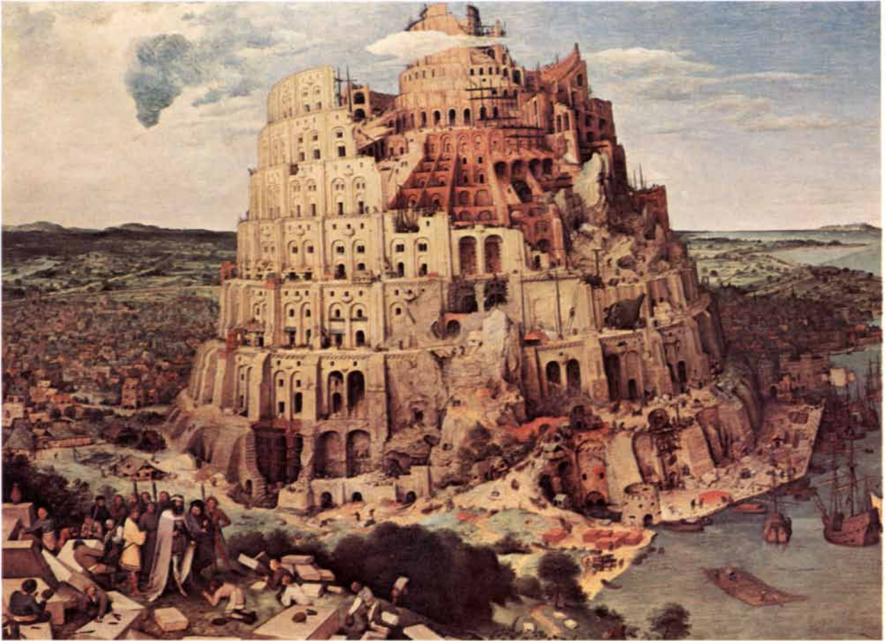
“TOWER OF BABEL,” painted by Pieter Bruegel the Elder in oil on an oak panel, depicts the Babel story told in the Book of Genesis and also shows a number of 16th-century construction techniques. They include the man-powered lifting devices on the right side of the tower
