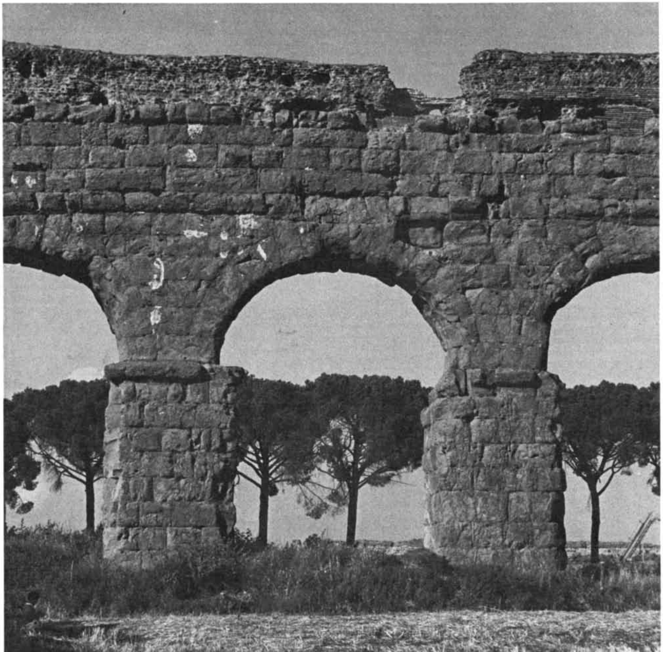
ARCHED BRIDGE carried two aqueducts a distance of 6.5 miles near Rome. The photograph shows part of the longest section still in existence, a length of some 1,500 yards including 153 arches. At this
