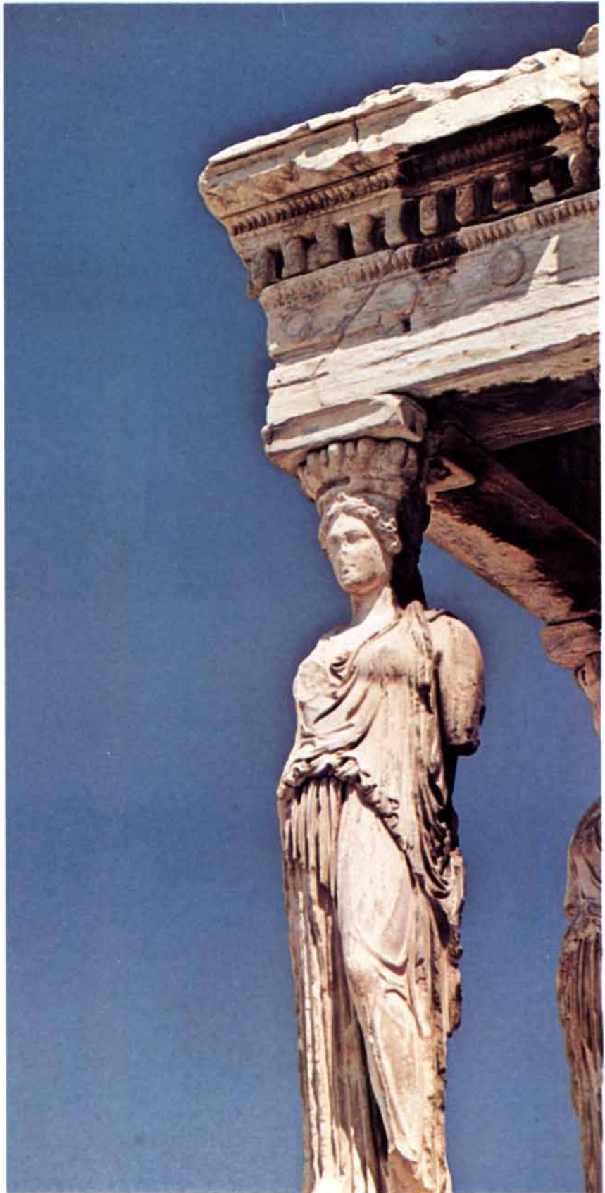
CARYATID FIGURE , one of six serving as supports for the porch roof of the Erechtheum on the Acropolis, shows the effects of 2,300 years of weathering. The marble has been damaged by sulfur dioxide, which built a coat of gypsum on the surface. Adjacent areas of the building have also deteriorated from rusting of iron reinforcing bars installed between 1902 and 1909.
