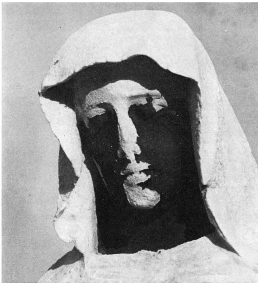
WEATHERED MADONNA stands in a cemetery in New York City. The weathering is the result of the reaction of the stone with oxides of carbon, sulfur and nitrogen dissolved in rainwater. In the open areas of the statue the reaction products have been washed off by rain in a natural cleaning process, but in the recessed and partly protected area of the face they have formed a crust that has begun to fall off in patches, aggravating the decay of the stonework.
