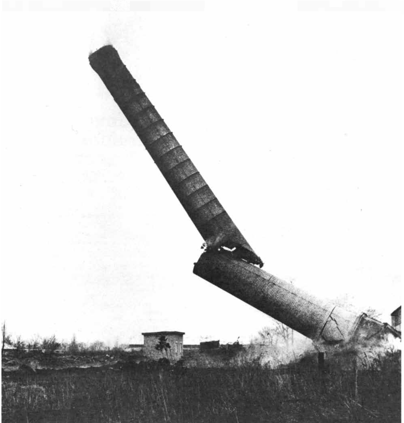
A chimney breaks as it falls
