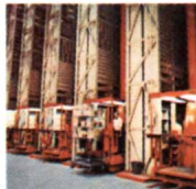
automated storage and retrieval systems...
