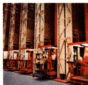
automated storage and retrieval systems...
