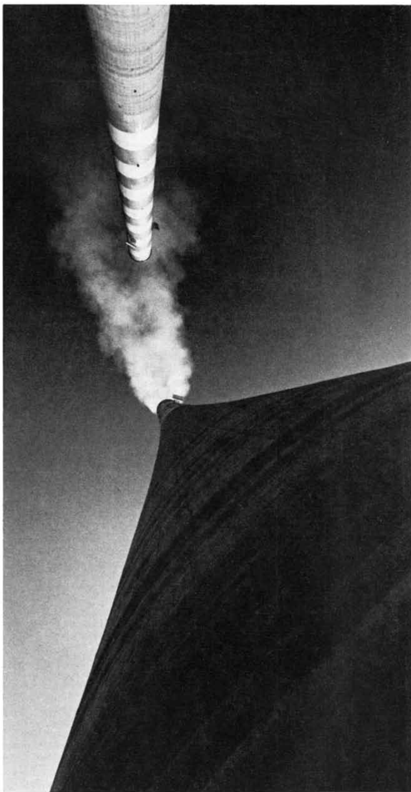
TALL STACKS of the generating station of the Tennessee Valley Authority in Cumberland City, Tenn., reach a height of 305 meters (1,000 feet). They typify a widespread trend to build taller stacks to reduce the concentration of sulfur and nitrogen oxides near the ground, since that is where the Environmental Protection Agency (EPA) and similar state agencies make measurements of such concentrations. By putting the oxides higher into the atmosphere, however, the stacks cause them to be carried farther, turning a local problem into a regional one.
