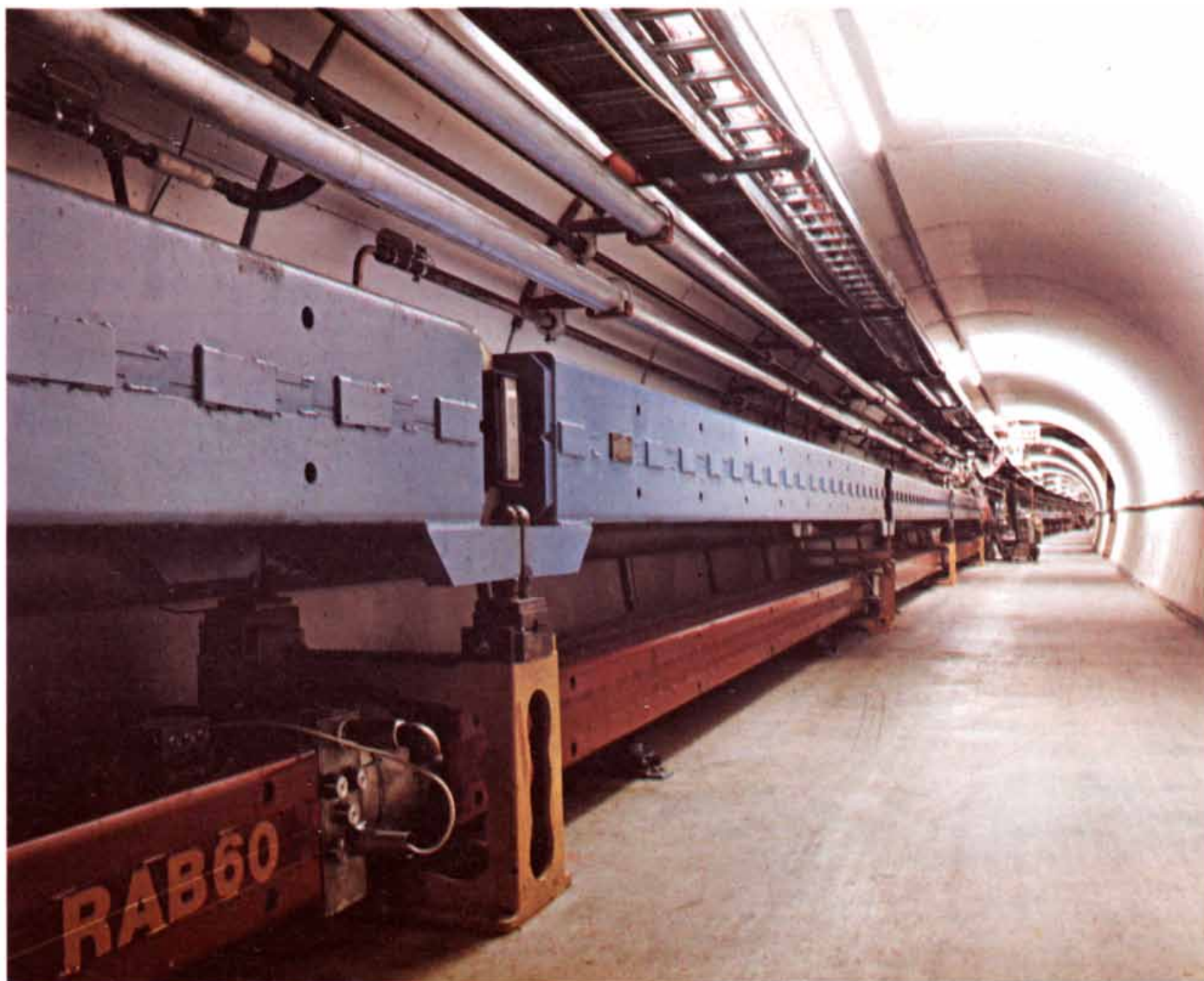
TANDEM ACCELERATORS occupy a single tunnel at the Fermi National Accelerator Laboratory (Fermilab) near Chicago. The blue objects in the upper tier are the beam-bending magnets of the original "main ring" proton synchrotron, which began operating in 1972 and has reached a peak energy of 500 billion electron volts (GeV).
