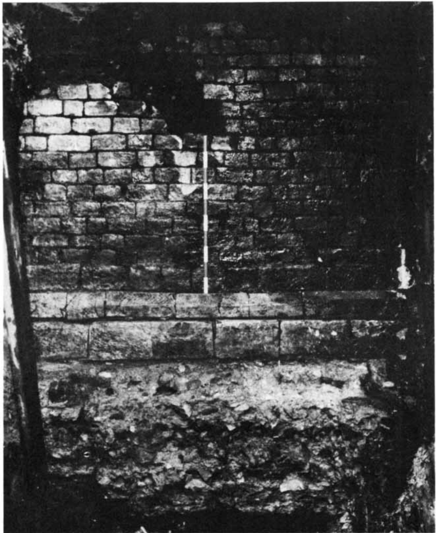
FORTRESS WALL , standing 16 masonry courses high above a chiseled plinth that is supported by a mortar-and-cobble foundation resting on oak piles, is another relic of Roman York uncovered by chance during commercial excavation for a deep sewer in the center of the city.
