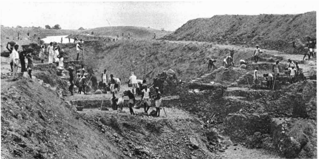
Earthworks excavation in India carried on by hand, hoe and woven basket.
