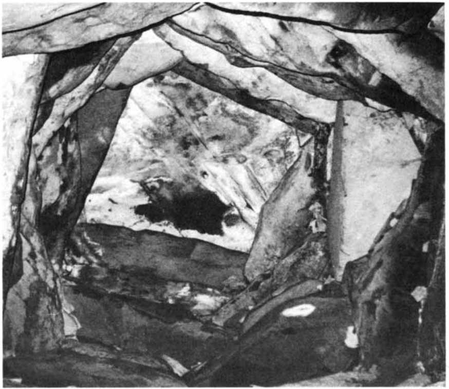
LOOKING UP to the top of the corbeled vault at Newgrange, this photograph reveals its stepped construction. Each successive layer of slabs was placed closer together until capstones could bridge the narrowed gap. A similar corbeled vault was built at Maes Howe in Orkney.
