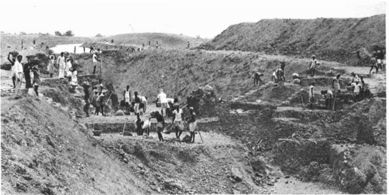
Earthworks excavation in India carried on by hand, hoe and woven basket.
