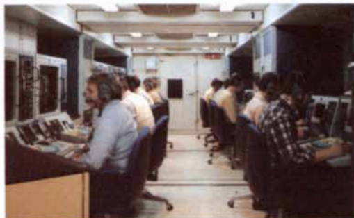
Automated signal processing and control system.
