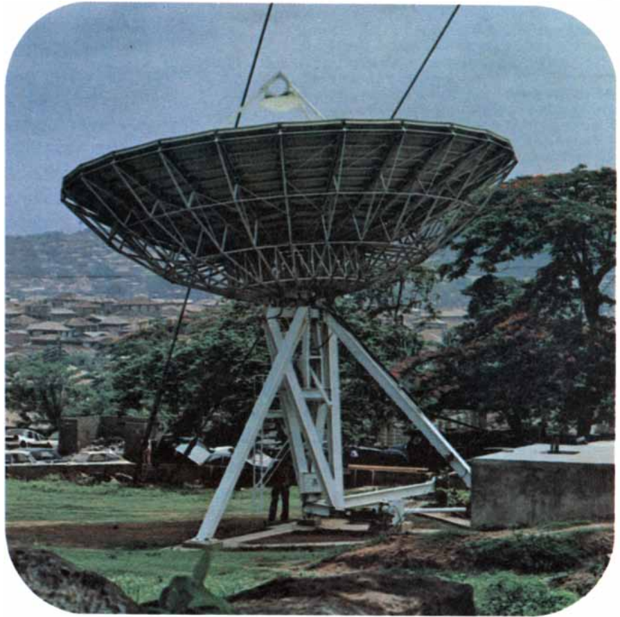
HARRIS satellite communication system terminal in Ibadan, Nigeria
