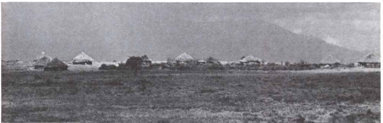
VILLAGE in the Monduli district of the Arusha region of northern Tanzania was settled in the mid-1970's as part of the government's program of "villagization." The walls of the houses consist of poles covered with clay and dirt. The roof is thatch. The floor and the foundation are clay and mud covered with a thin layer of cow dung, which
