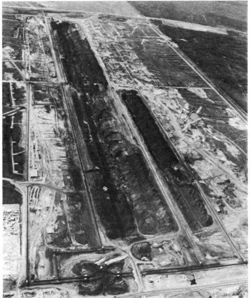
TAR SANDS OF ALBERTA are exploited by means of surface-mining techniques. Seen here are two of the trenches excavated in a tar-sand deposit by Syncrude Canada Ltd. Draglines pile up the tar-bearing soft rock in windrows; two can be seen at work close to the near ends of the trenches. The rock is then transferred to conveyor belts by means of bucket-wheel reclaimers; one can be seen at work just above the left dragline. The long conveyor belts deliver the rock to the processing plant (not seen), where the tar is converted into synthetic crude oil.
