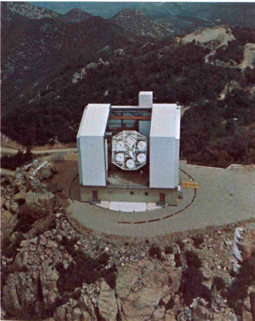
MULTIPLE-MIRROR TELESCOPE (MMT) on Mount Hopkins in Arizona was used to make measurements of the twins' red shift. Each of the six mirrors is 1.8 meters in diameter.
