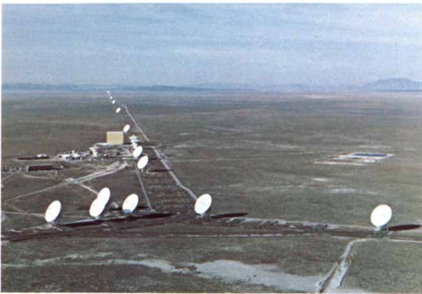
VERY LARGE ARRAY (VLA) that produced the display on the preceding page is a Y-shaped collection of 27 dish antennas near Socorro, N.M. Each of the dishes is 25 meters in diameter.
