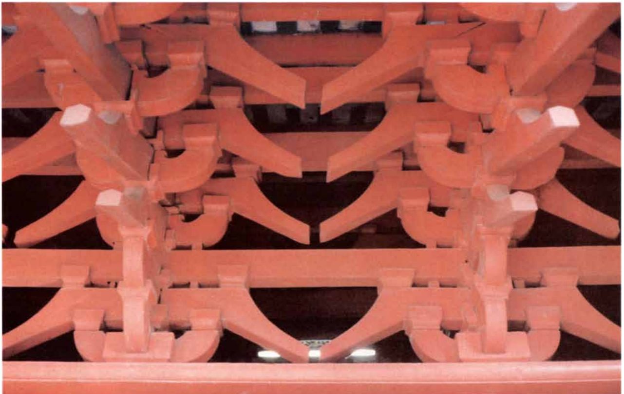
BRACKET-ARM ARRAY , seen from below, rises repetitively to support the roof beams of another building in the same temple com-
