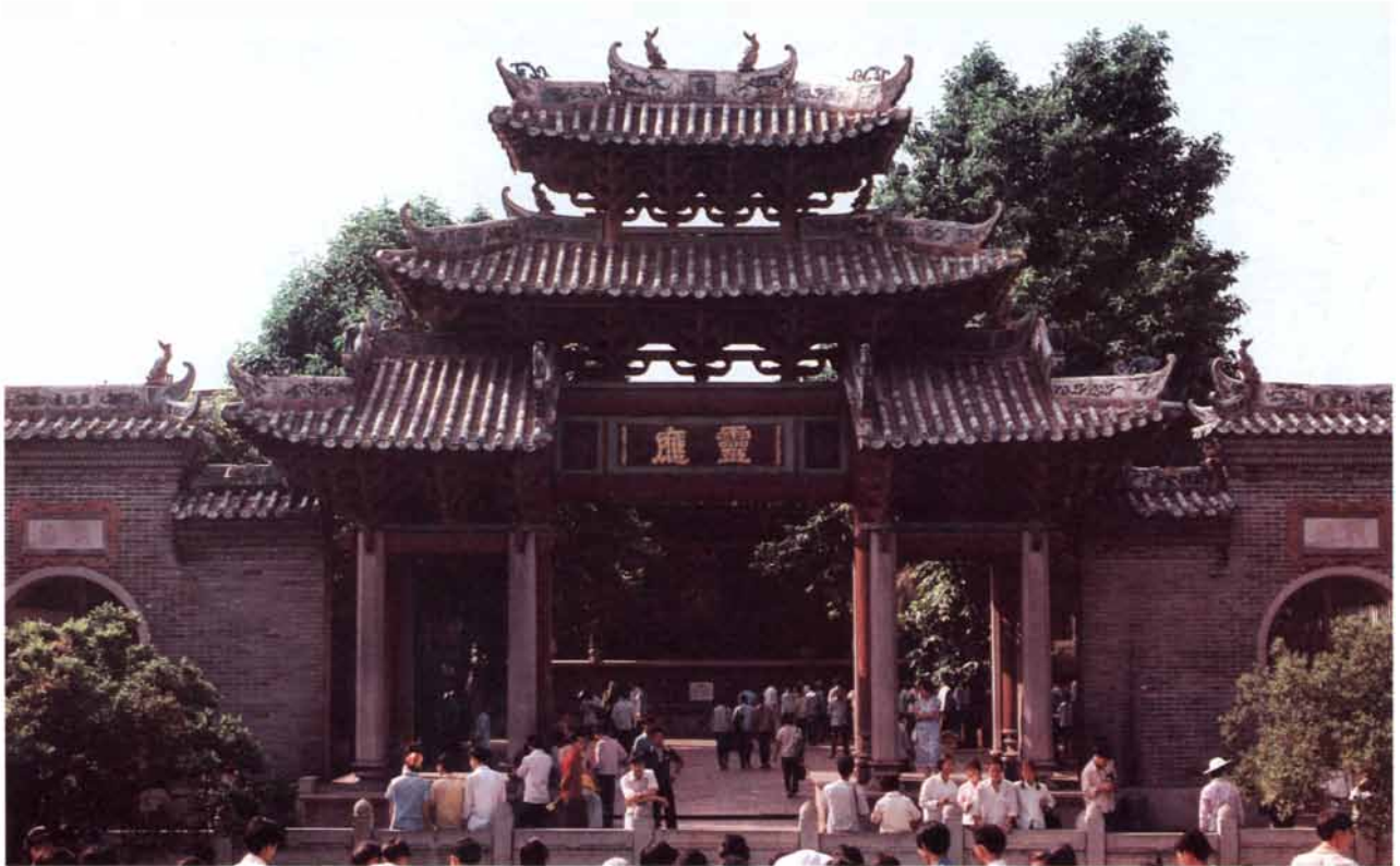
THREE-TIER ROOF of a temple gateway near Canton is supported by 12 columns. The load of each roof component is distributed to the columns by means of a series of corbeled sets of bracket arms,
