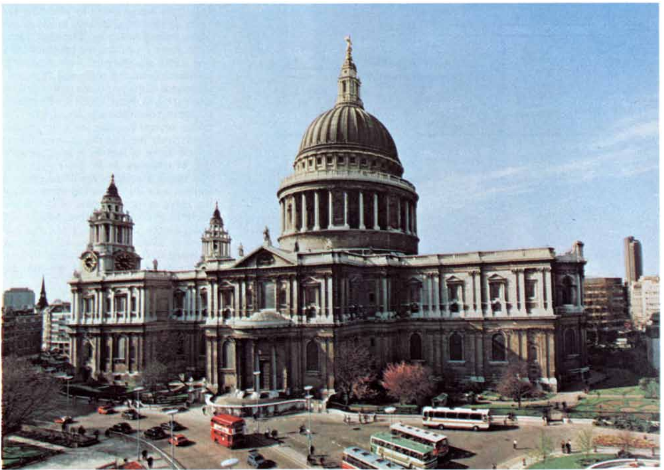
ST. PAUL'S CATHEDRAL looks today almost as it did when Wren built it. The balustrade was added over Wren's protest in 1717, when
