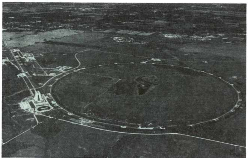
The Fermilab accelerator, a four-miles in circumference tunnel, dwarfs the Fermi National Accelerator Laboratory office and laboratory building (left) though the building towers far above the Illinois plain near Batavia. Protons accelerate in the ring to near relativistic velocities, then go to the experimental areas at the extreme left just above the office building. Facility gets $10 million worth of electric power each year over lines leading toward upper left.
