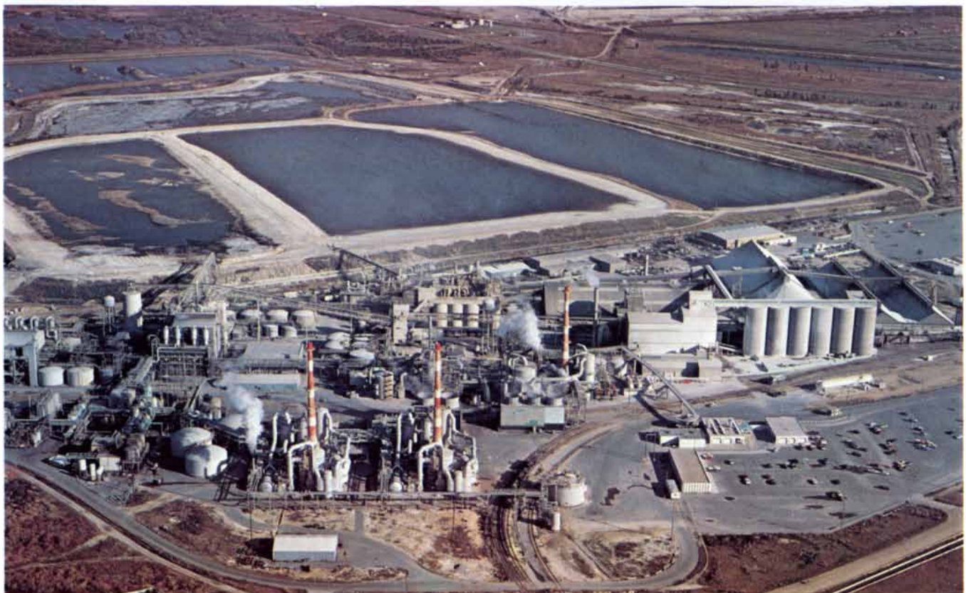
FERTILIZER PLANT of W. R. Grace & Co. near Bartow is where beneficiated phosphate rock is made into granulated fertilizer. The six silos at the right store the finished product; the material piled be-
