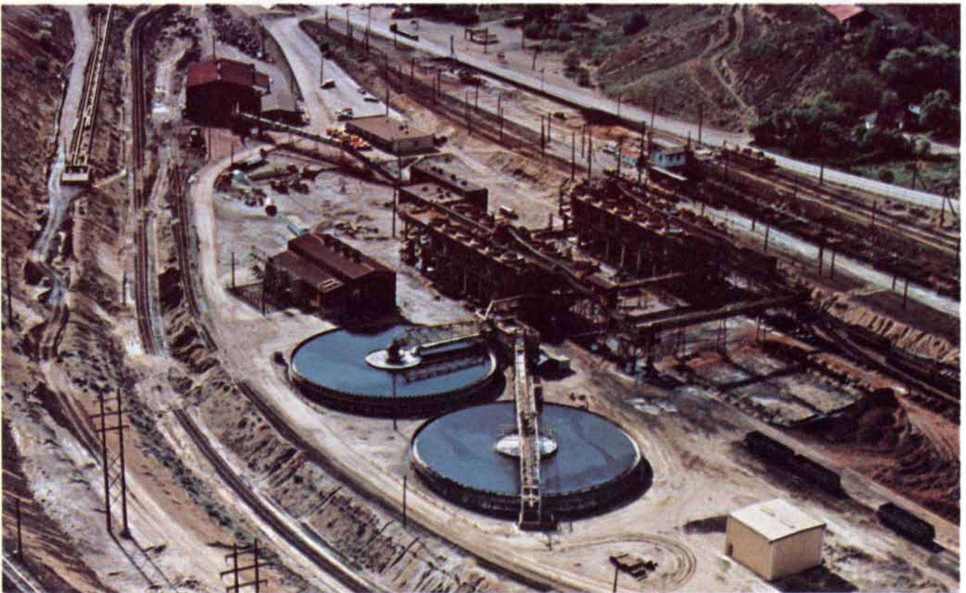
PRECIPITATION PLANT removes copper from the leaching solution by a cementation reaction, in which ferrous iron replaces the copper in solution. Here scrap iron is used to precipitate the copper in two modules; each module consists of 13 units called precipitation
