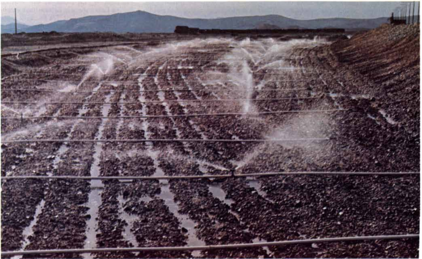
LEACHING SOLUTION is sprayed by a sprinkler system on top of a copper-leaching dump similar to the ones shown on the preceding
