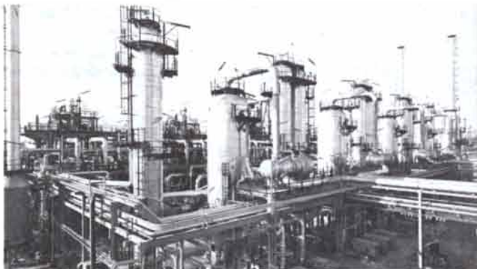
Methane-Reforming Plant – Part of the World's largest Oil-from-Coal-Plant.
