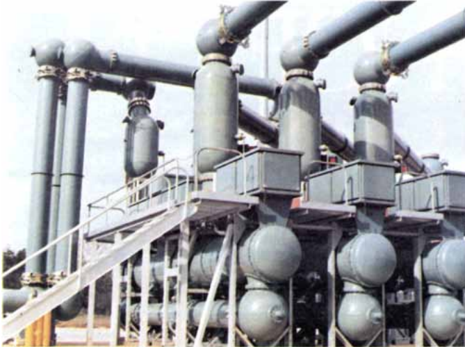
The most powerful electrical networks, 800,000 Volts switchgear in the United States.
