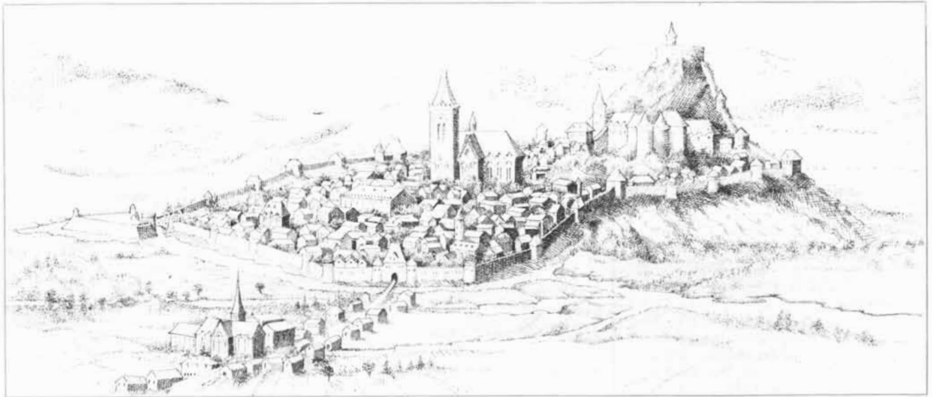
FORTRESS BOURG OF RETHEL in the Ardennes, depicted in another drawing after a 15th-century engraving, had also grown from a motte-and-bailey castle. By then both the motte and the bailey had been faced with blocks of chalk and surrounded with a stone wall
