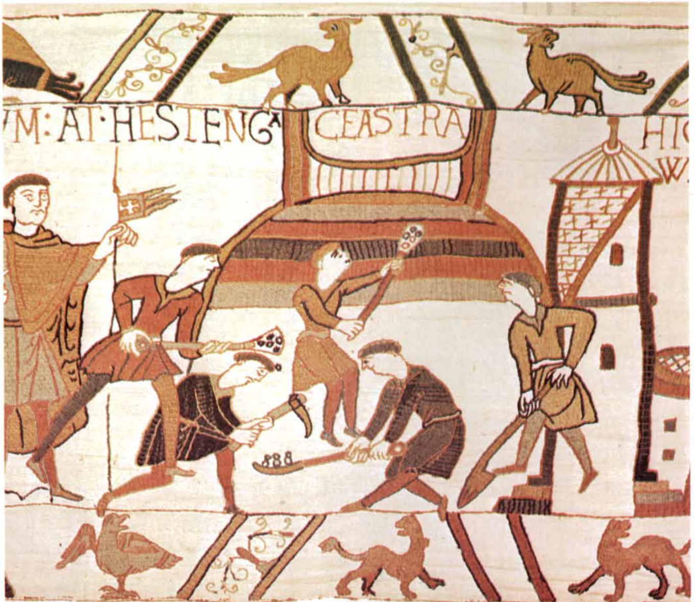
MOTTE AT HASTINGS , the site of William the Conqueror's battle with Harold, appears in a detail from the Bayeux tapestry. The corner posts of the tower have been put up and are being covered
