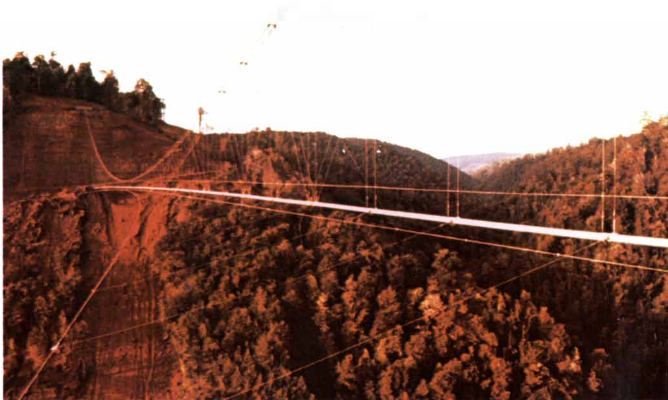
IRON-ORE-SLURRY PIPELINE crosses a gorge of the Savage River in northwestern Tasmania. It carries ore concentrate from the
