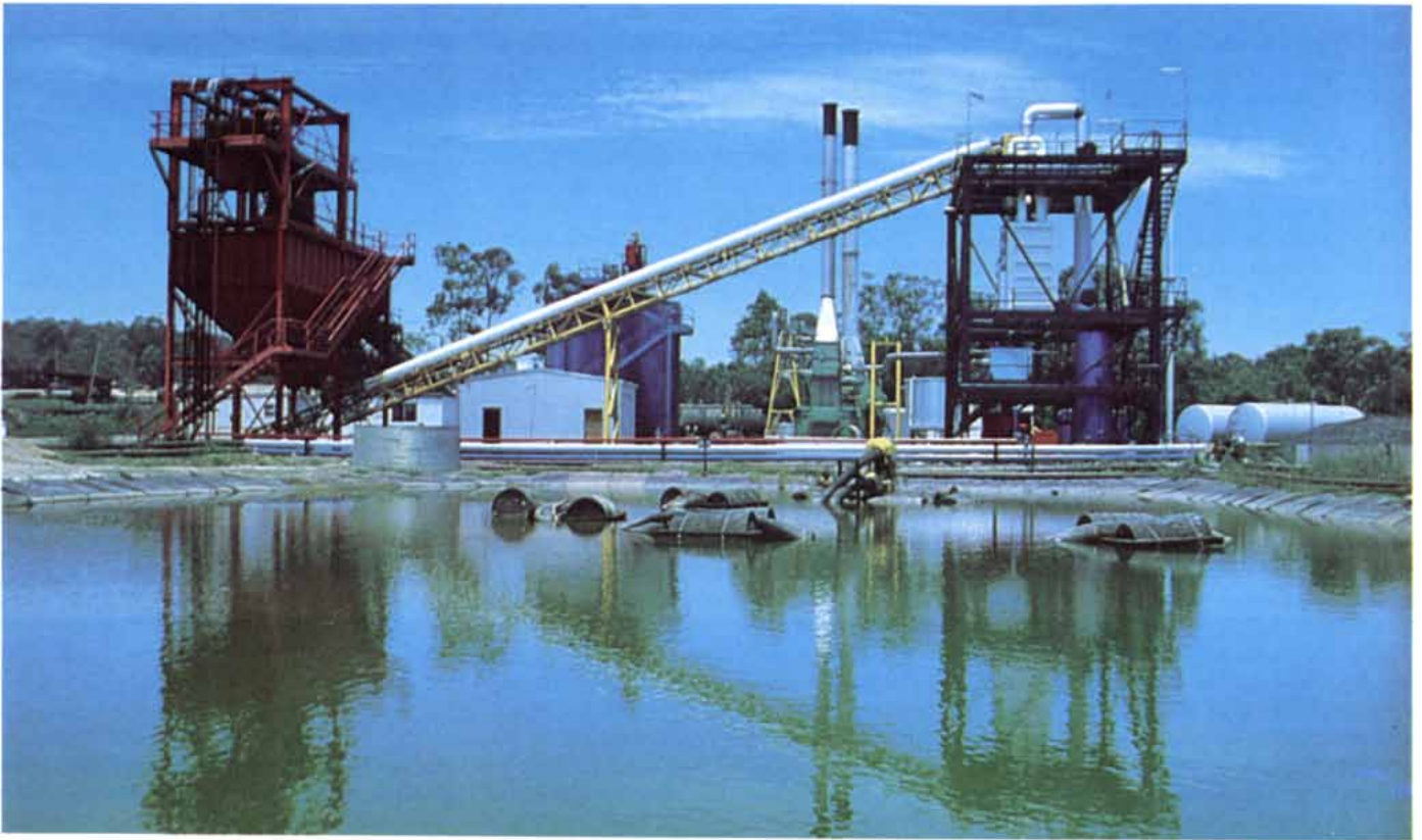
The 30 ton per hour pilot plant at Stockton Borehole Colliery, Taralba, New South Wales.
