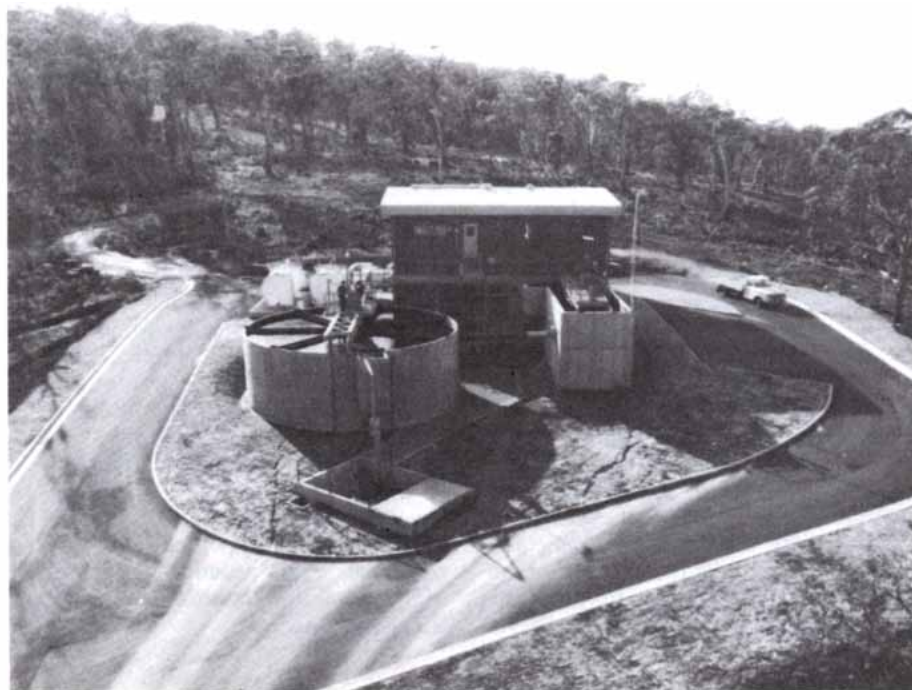
The Sirofloc plant at Bell Bay, Tasmania is compact and produces 5,280,000 gallon/day of treated water. Major equipment includes contact tanks (left) and clarifier (right).
