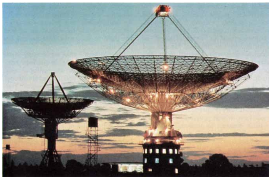
The 64-meter Parkes radio telescope, New South Wales, was constructed by CSIRO in 1961.
