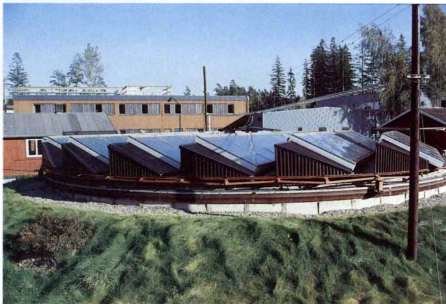
Studsvik Energiteknik's experimental solar-heated hot water basin. The solar panels sit atop an insulated tank filled with solar-heated water for heating the office building in the background.
