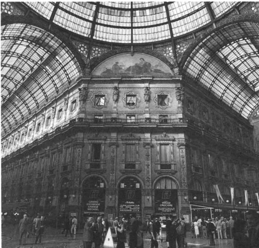
GALLERIA VITTORIO EMANUELE was inspired by the Crystal Palace. As in the Palace, broad interior spaces and large expanses of glass contribute to a sense of openness and light.
