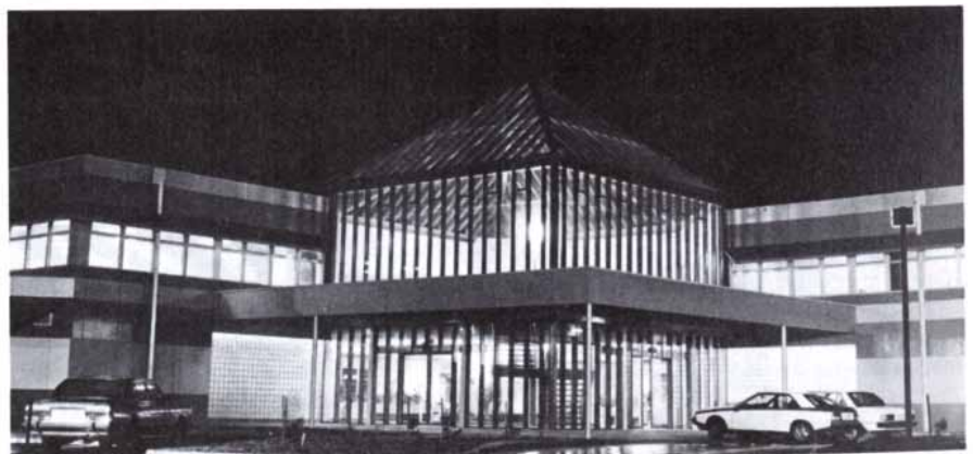
Innovation House, Technology Park, Adelaide, South Australia
