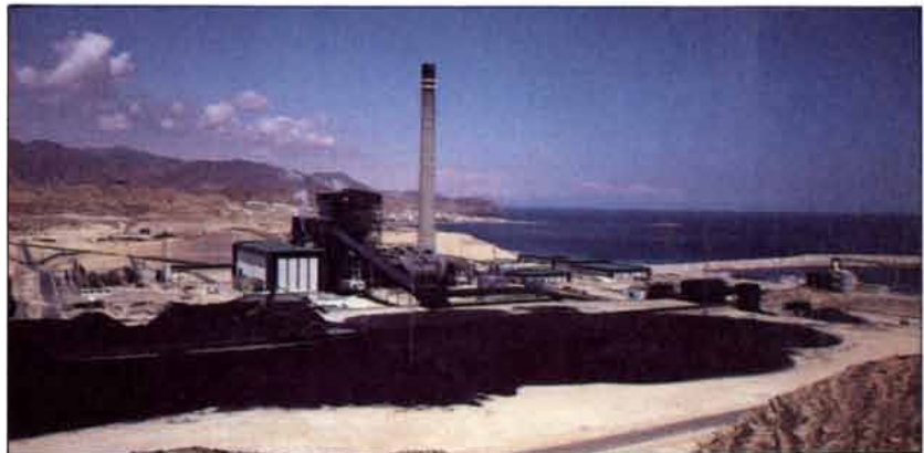
ENDESA's new coal-fired power station at Carboneras.
