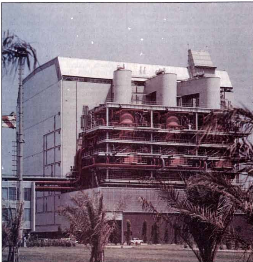
The nuclear power station at Latina, south of Rome.
