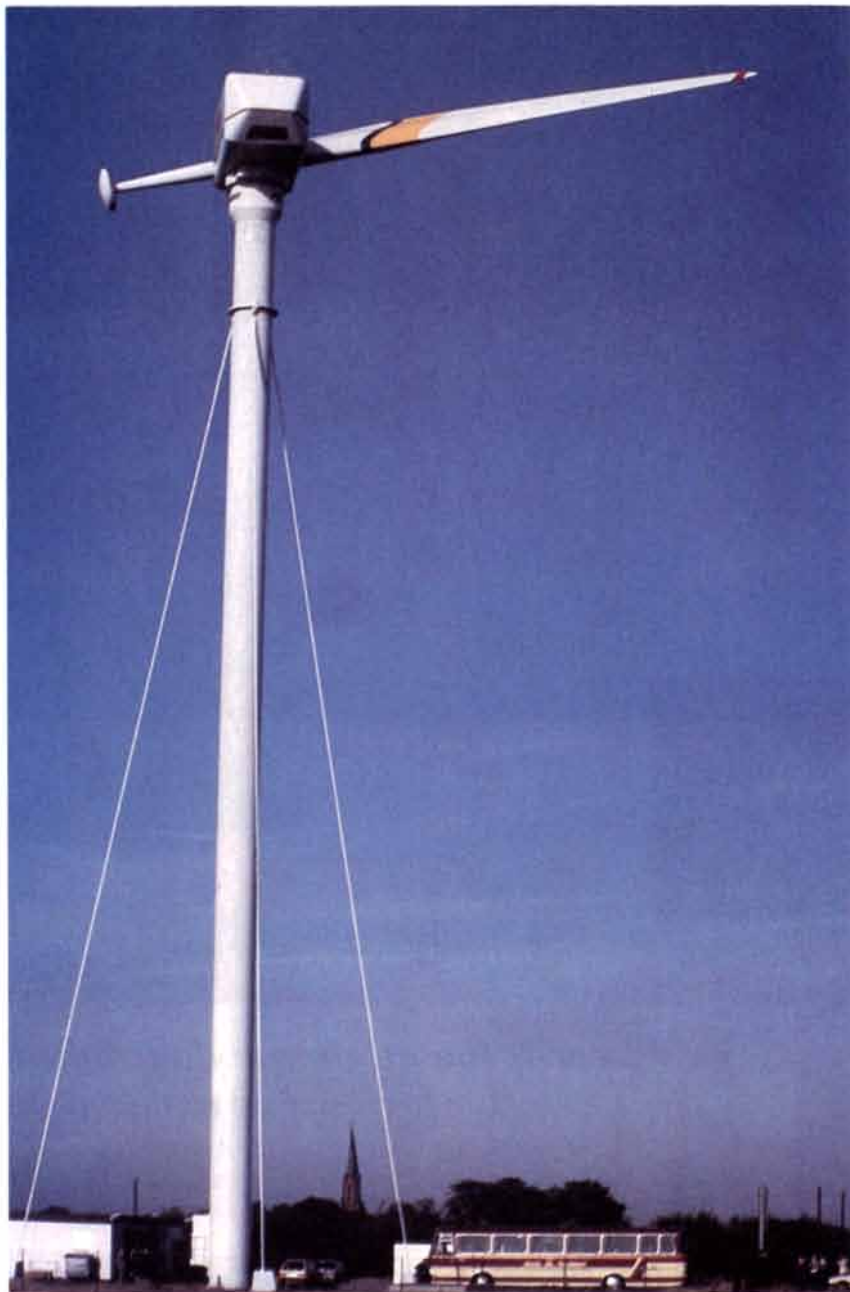
SINGLE-BLADE WIND TURBINE called Monopteros is an experimental structure near Bremerhaven in West Germany. It represents the kind of novel configuration that turbine designers have tested in the quest for higher speed, reduced blade area and lower cost.
