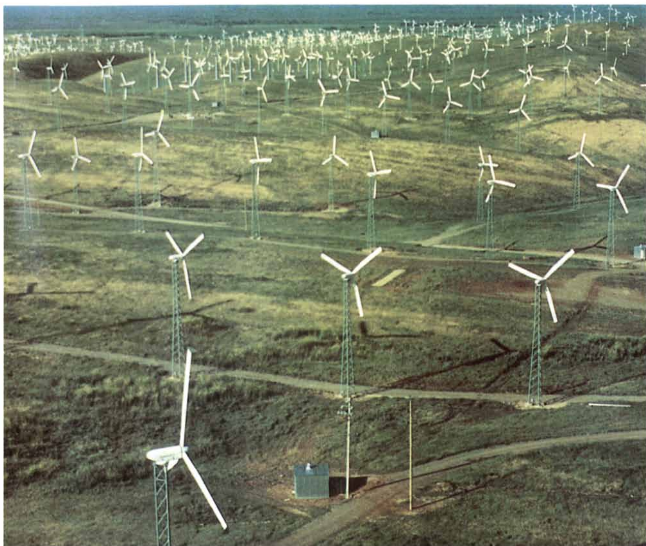
WINDMILL FARM in California consists of an array of wind turbines contributing to the local power grid. More than 13,000 tur-
