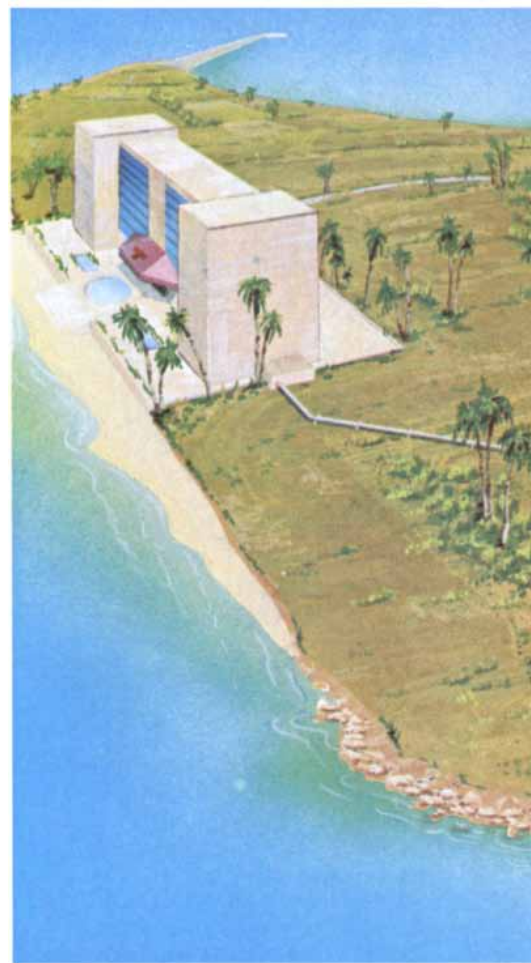
INTEGRATED SYSTEM based on ocean thermal-energy conversion (OTEC) is depicted. An electric power plant has three large pipes running out to the sea: a warm-
