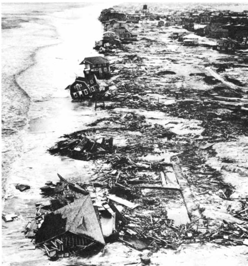
STORM DAMAGE is a hazard for buildings near the shoreline. This is how the shoreline of Fire Island, N.Y., looked not long after the Ash Wednesday (March 7) storm of 1962, a particularly severe northeaster. Such a major storm occurs about once per century.
