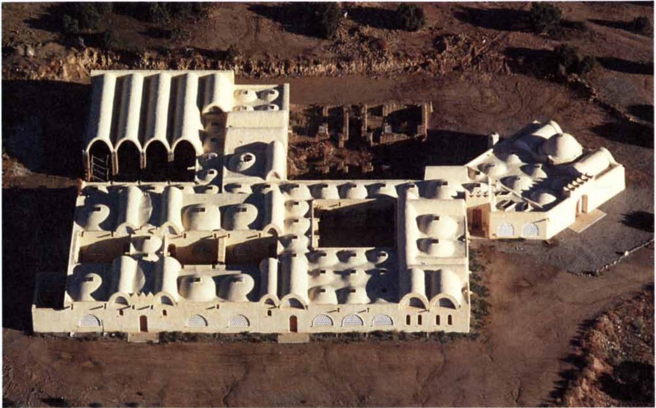
MODERN MUD-BRICK VAULTS built in the traditional way support the buildings occupied by the Dar Al Islam educational foundation at Abiquiu in New Mexico. The complex was designed by the Egyptian architect Hassan Fathy. The structure projecting to the right is a mosque. The remainder of the complex is a school; the unfinished structure at the upper left will house the cafeteria.
