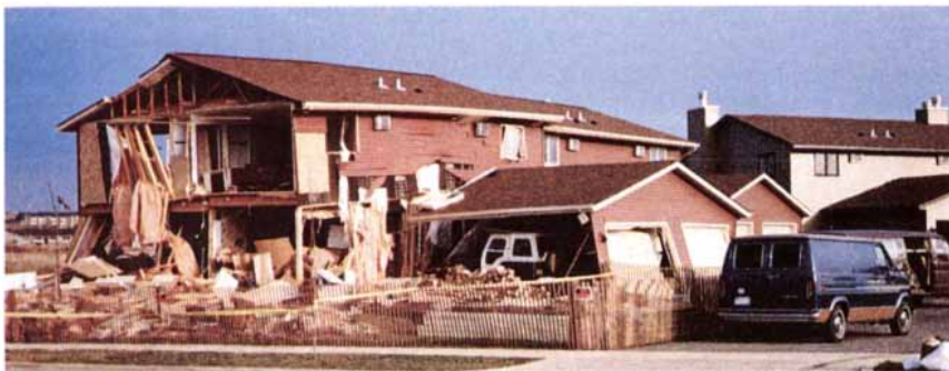
TOWNHOUSE EXPLODED across the street from a closed landfill in Madison, Wis., on November 19, 1983. Methane produced by the decomposition of solid waste seeped underground into the house and was ignited. Two tenants were burned in the explosion. Since the accident a methane-control system has been installed.
