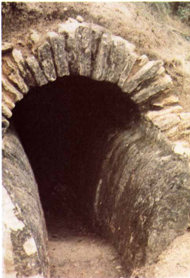
SURVIVING SEGMENT of the water channel (left), now encrusted with calcium deposits, is typical; most of the conduit ran underground and had a similar shape. The area meant to hold water was usually 1.2 meters square; the total height of the
