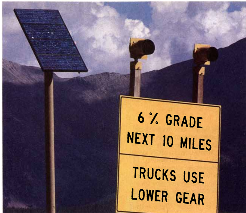
SIGN OF THE TIMES on a mountain highway has lights powered by photovoltaic cells. The price of the cells has dropped rapidly, thereby expanding their market. Time can be gained to research and develop such innovative technologies, which increase energy supplies, by consuming existing energy resources more efficiently.
