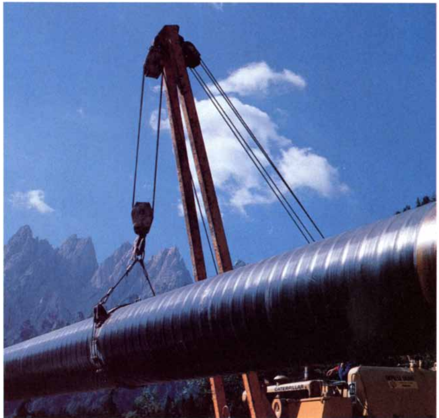
Doubling the methane pipeline, USSR-Italy
