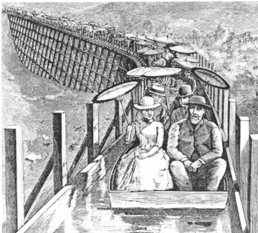
Floating down a trestle on the San Diego flume
