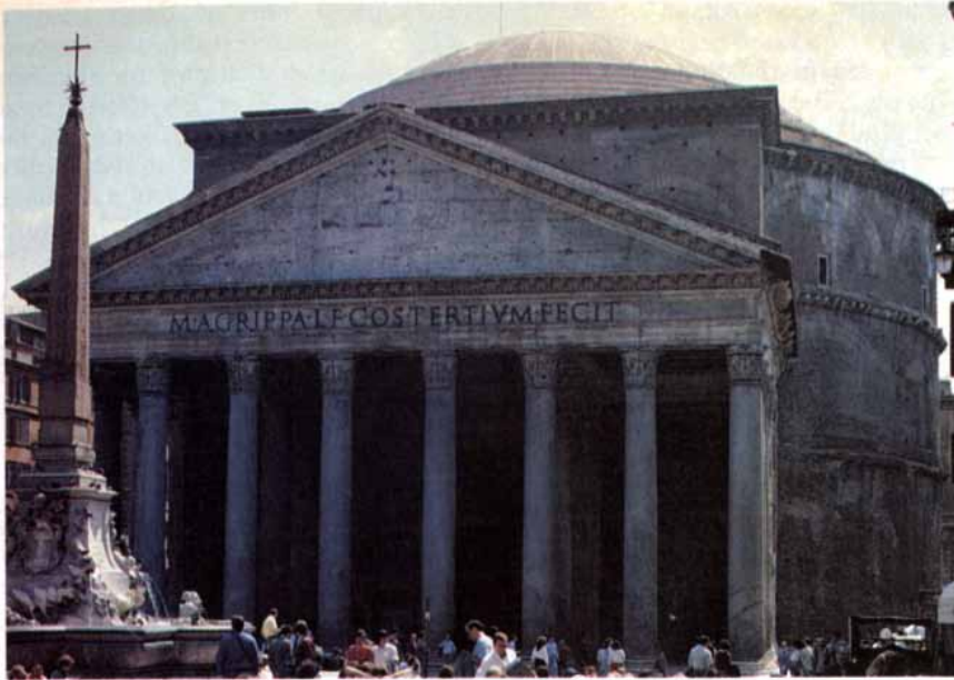
PANTHEON in Rome was one of the buildings that Filippo di Ser Brunelleschi, architect of the cupola of Santa Maria del Fiore, studied. It has a circular dome and an oculus, or eye, at the apex, the only source of natural light for the interior.
