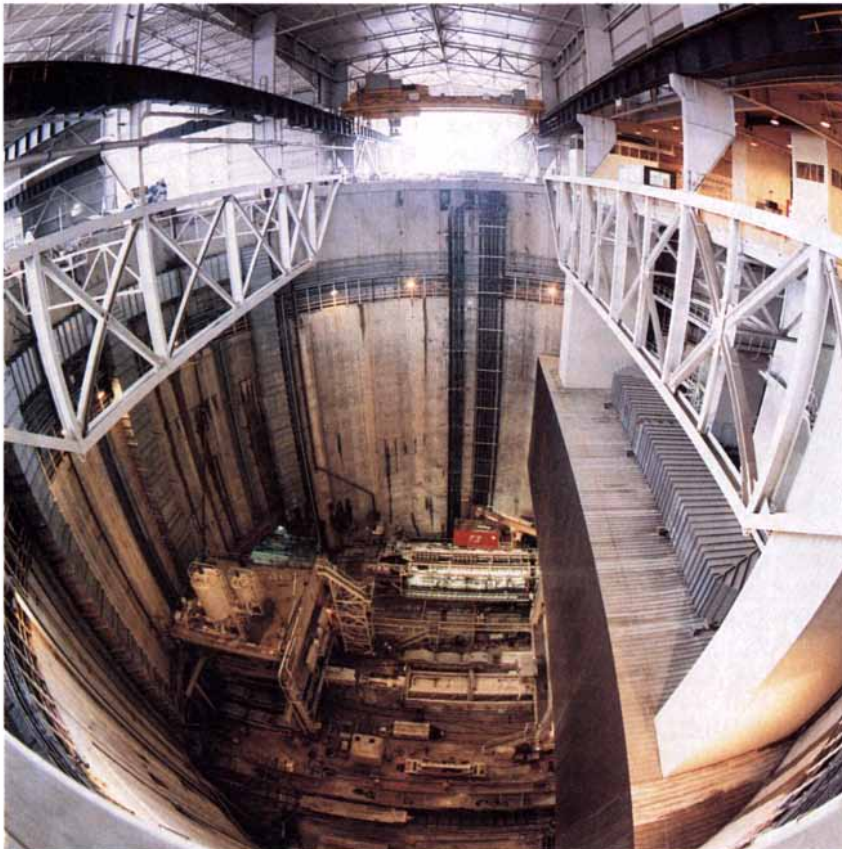
The access shaft in Sangatte, France. QA Photos.
