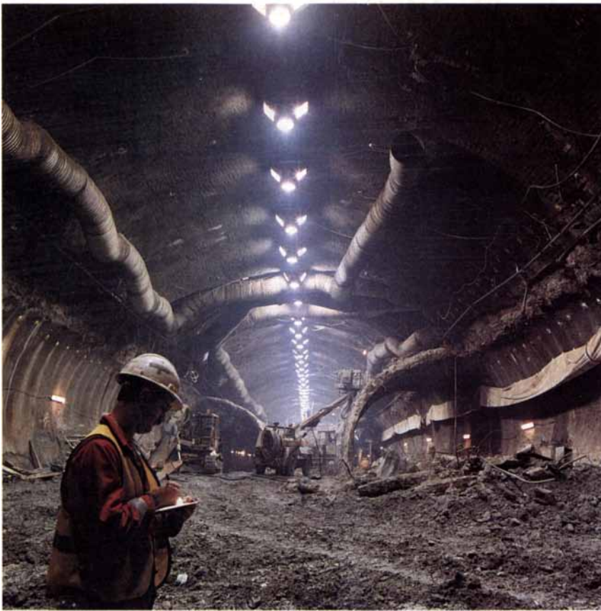
Newly excavated section of the running tunnel. QA Photos.
