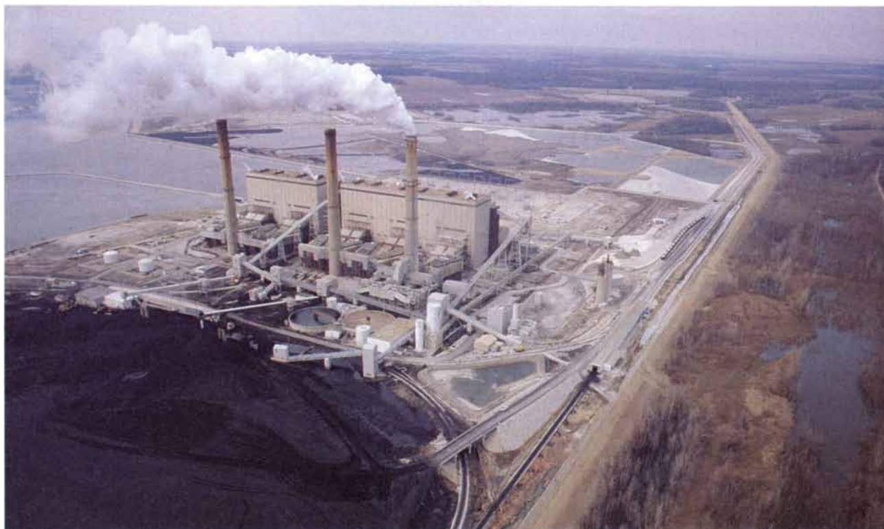
GIBSON GENERATING STATION in southwest Indiana is bordered by a 3,000-acre artificial lake and a 160-acre wildlife preserve, both of which were built by the utility. Flue gas
