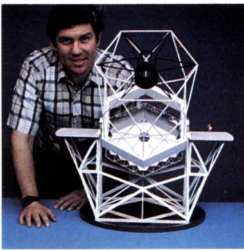
KECK TELESCOPE uses a segmented-mirror design proposed by project scientist Jerry Nelson ( left ). In 1987 workers began assembling the telescope's dome. Two years later they installed the telescope structure; in October 1990 the first
