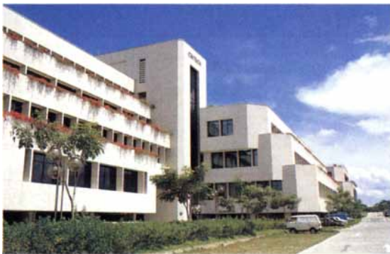
View of CINTECH, the Center for Information Technology
