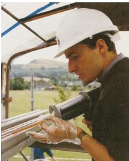
BRIDGE OVER THE RIVER TAY was built last year in Aberfeldy, Scotland, from glass fiber-reinforced composites. Components of the footbridge's deck were glued together ( bottom left ), and then the deck was winched over the two A-frame towers by a student. The project demonstrated an advanced composite civil structure.
