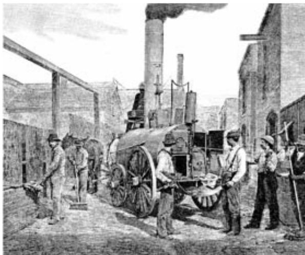
Traveling garbage burner of Chicago
