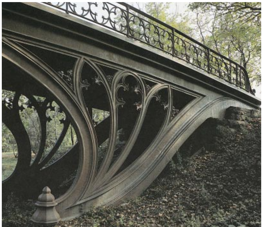
CAST-IRON ARCH BRIDGE in New York City's Central Park, designed by Calvert Vaux and Jacob Wrey Mould, was constructed in 1864.
