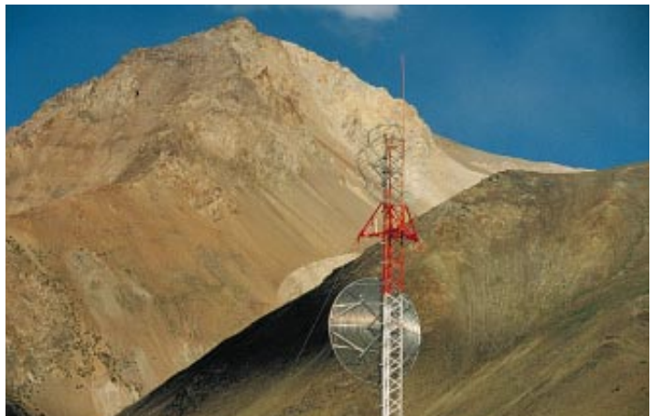
PARTS OF ARGENTINA inaccessible to wire-line telephone service are now served by a wireless network built in less than six months.
