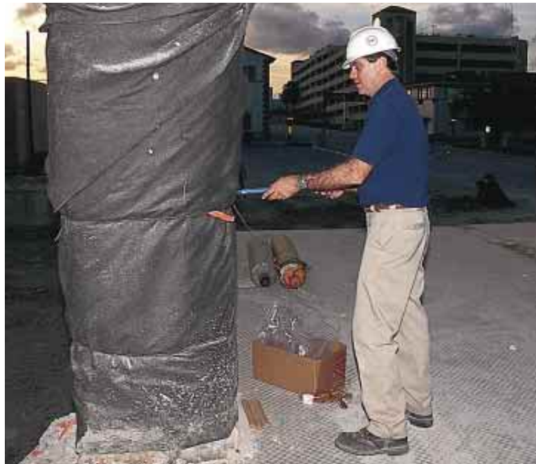
LOADING OF COLUMNS with dynamite required holes to be drilled by a vehicle outfitted with a rotary drill ( top left ). Later, sticks of dynamite were broken, and blasting caps were inserted ( bottom left ). The primed dynamite was packed, cushioned by small sandbags, into the holes with a wooden dowel ( wielded by Doug at top right ).
