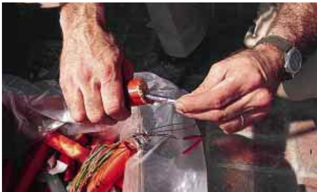
LOADING OF COLUMNS with dynamite required holes to be drilled by a vehicle outfitted with a rotary drill ( top left ). Later, sticks of dynamite were broken, and blasting caps were inserted ( bottom left ). The primed dynamite was packed, cushioned by small sandbags, into the holes with a wooden dowel ( wielded by Doug at top right ).
