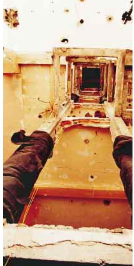
COLUMNS WERE WRAPPED with chain-link fencing and then heavy fabric (left) to prevent debris from flying everywhere. Once the columns were loaded with dynamite, wires from the blasting caps in each column were connected to one another. Finally, wires from the upper floors were dropped through an elevator shaft (right), drawn outside and connected to a blasting machine that set off the implosion.
