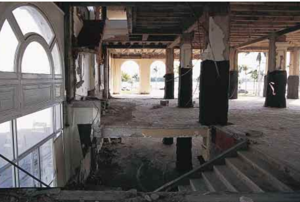
COLUMNS WERE WRAPPED with chain-link fencing and then heavy fabric (left) to prevent debris from flying everywhere. Once the columns were loaded with dynamite, wires from the blasting caps in each column were connected to one another. Finally, wires from the upper floors were dropped through an elevator shaft (right), drawn outside and connected to a blasting machine that set off the implosion.
