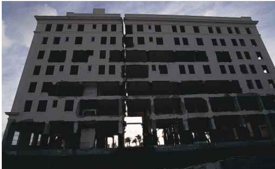
PREPARING THE HOTEL for implosion included slicing the building in two ( above, showing a back view ). This maneuver later helped to cause the north and south wings to collapse toward the center. In addition, steel cables were connected from one column to another ( top left ) to help draw the south wing of the building away from a narrow alley separating the hotel from a nursing home. A test blast done several days before the implosion assessed the structural integrity of the columns ( bottom left ) and showed their concrete to be rather weak.
