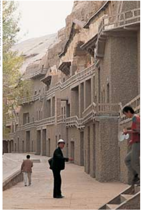
ENCROACHING SAND threatens the Mogao Grottoes (above) as it pours over the cliff face. The reinforced concrete facade (right), built in the 1960s, strengthens some of the grottoes that have been eroded by wind and weakened by earthquakes. As the map of the Silk Road (below) shows, Dunhuang sat on the very outskirts of China, at the point where the two arms of the trade network joined after circling the deadly Takla Makan Desert.
