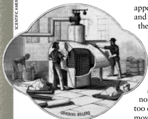
Asbestos used as insulating material
