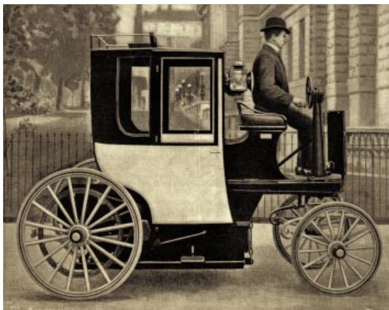
The new electrical cab
