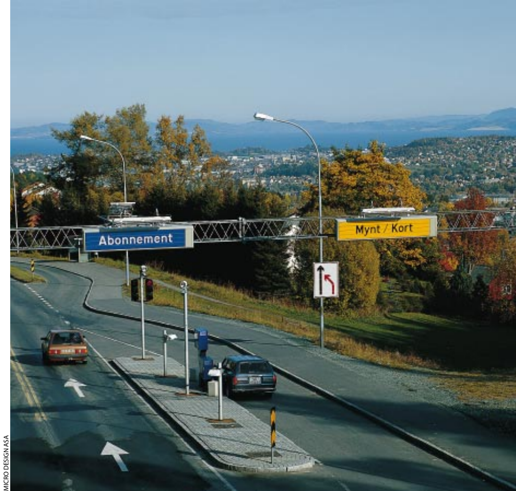
ELECTRONIC TOLLBOOTH s in Trondheim, Norway, allow cars to zip through without stopping. Radio transceivers collect the fees, which rise during rush hours. Such congestion pricing might ease chronic traffic jams elsewhere.
